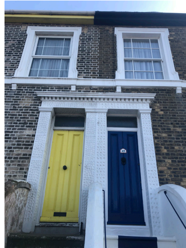
Decorative door frames
