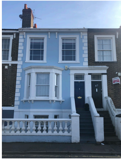
Decorative brackets under eaves
