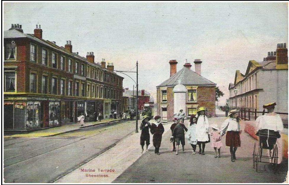
View of Neptune Terrace on right before the sea defence wall was built.
